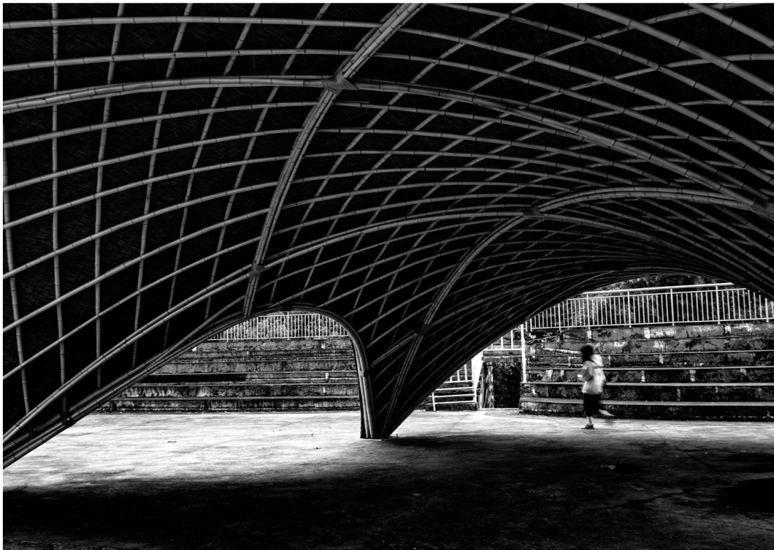
Figure 1. Interior view of Bamboo Canopy. Photographed under commission by the authors.
